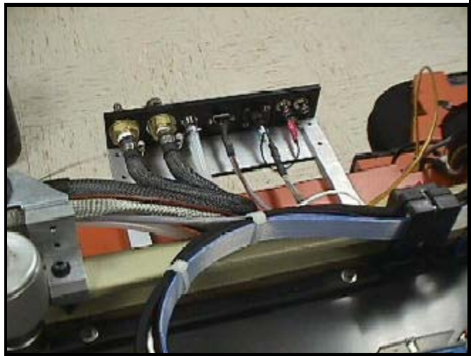
Figure 14 – Rear of hose connection plate
